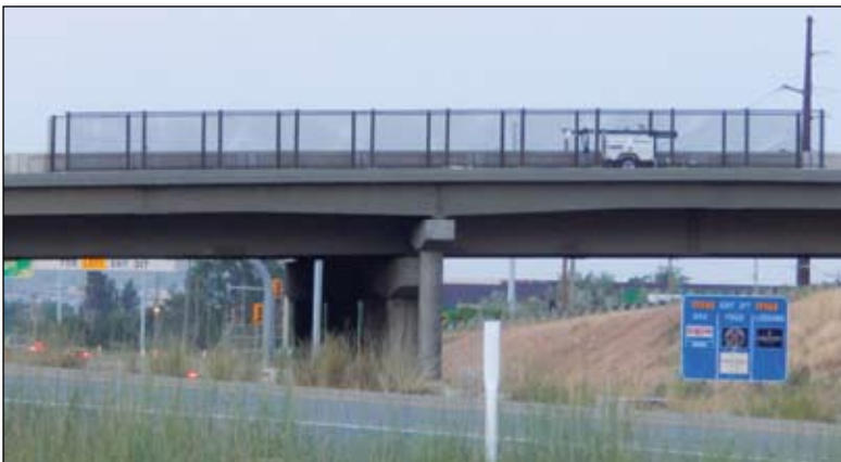
The pedestrian bridge fence on Parrish Lane over I-15 is expected to be completed soon.
